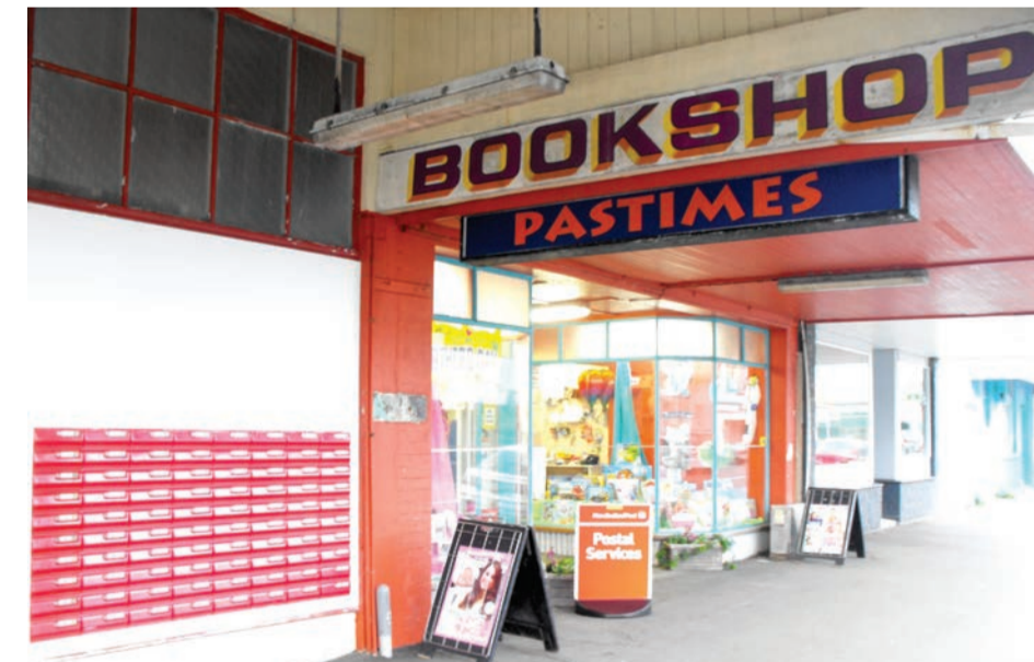
Pilot Computing which was next door to Pastimes and where the new post office boxes will be, has moved several doors further up the street into the old BNZ building beyond Four Square 45.
